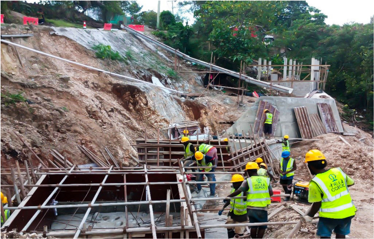
Retaining wall under construction at the Solomon Power site, part of the Auki Road Rehabilitation Project.
